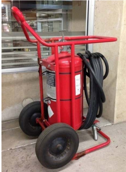
Picture 24. CAFS fire extinguisher with pressure bottle.
